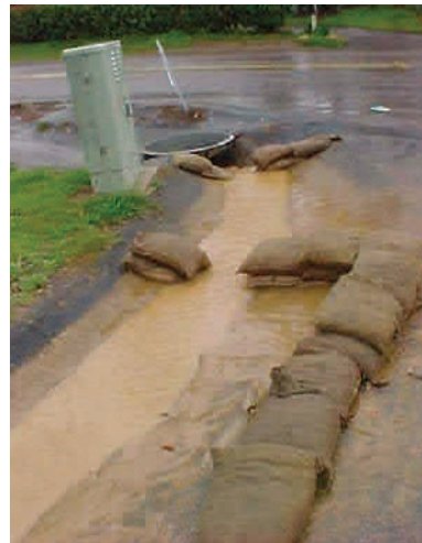
Figure 5. Make sure storm drain inlets are protected.
