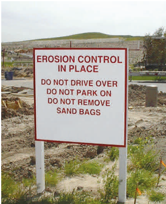
Figure 4. Use signage to help educate construction staff.
