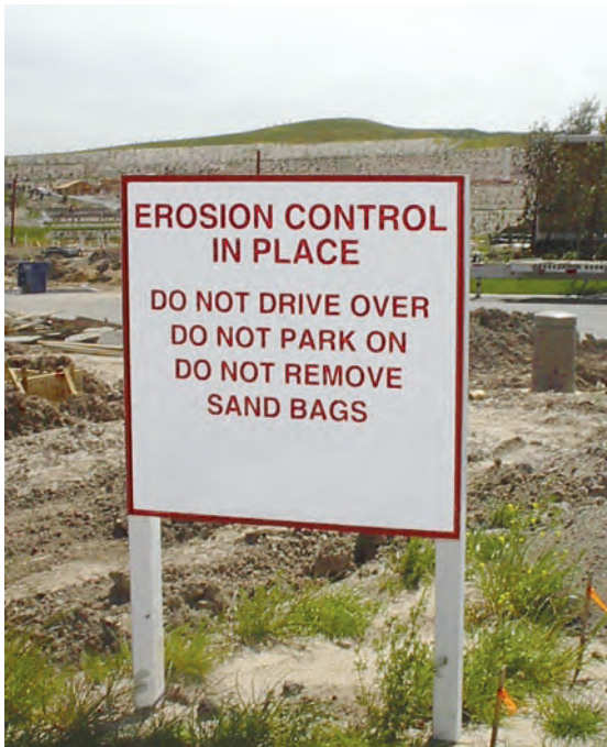
Figure 4. Use signage to help educate construction staff.
