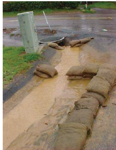
Figure 5. Make sure storm drain inlets are protected.
